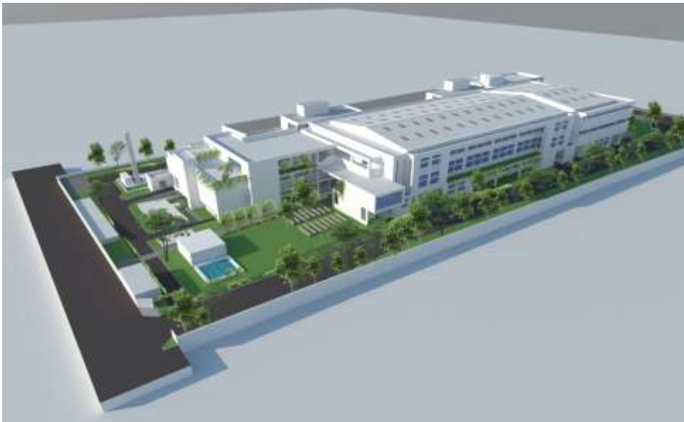
Integrated Eyewear facility - Chikkaballapur
