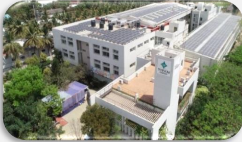
Manufacturing facility at Chikkaballapur
