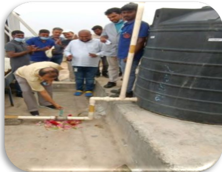
Ground water recharge Renovation
