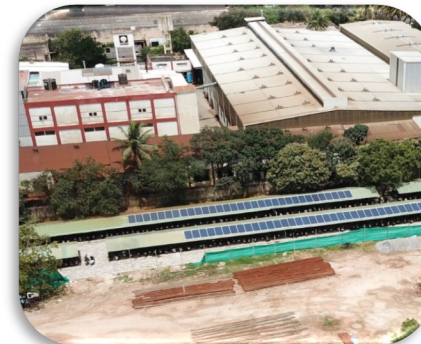
30KW Rooftop Solar Jewellery Factory
