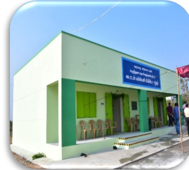
Classroom support Govt. school in Urigram
