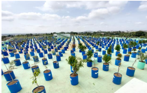
Oxygen roof garden over new building
